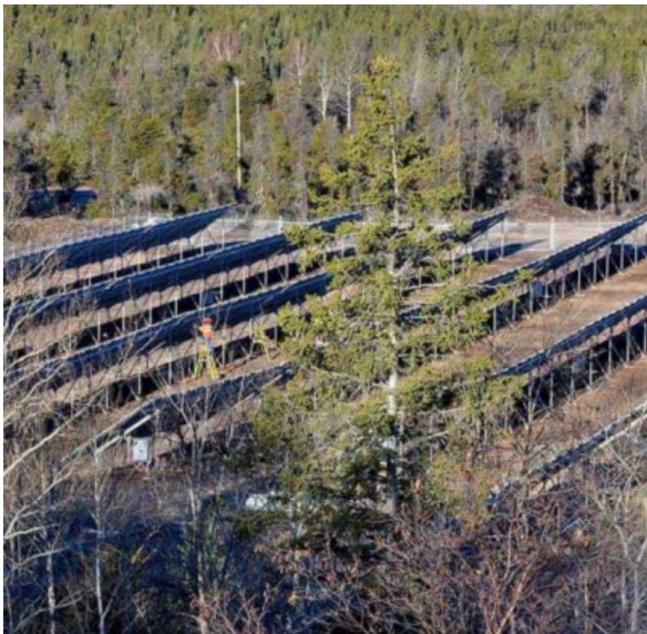
3NE Solar Panels
