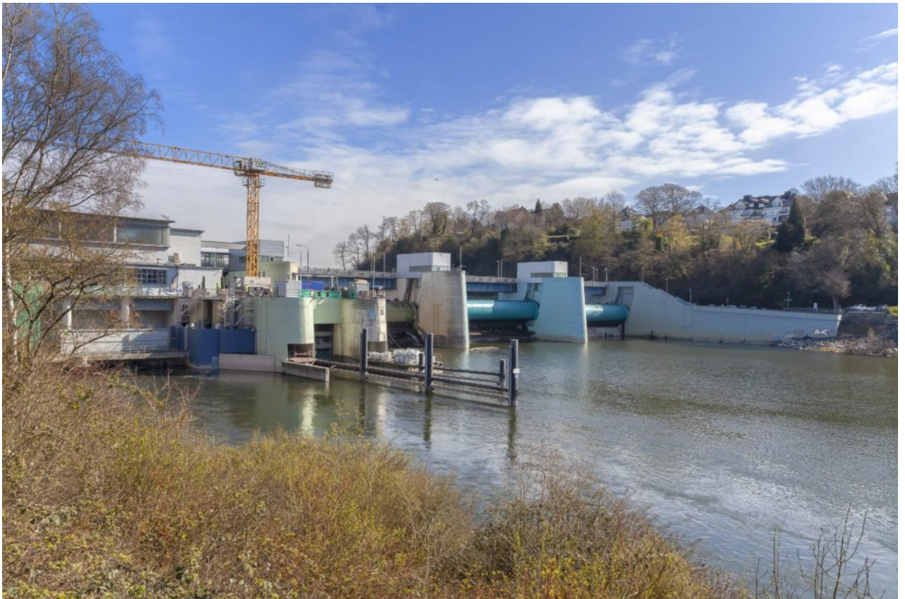
Fischliftsystem Baldeneysee / Fish Lift Mechanism Lake Baldeney
